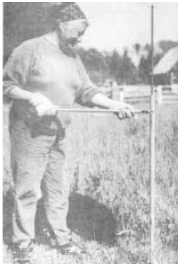
Marta Deak guides rebar fence posts into the ground.
