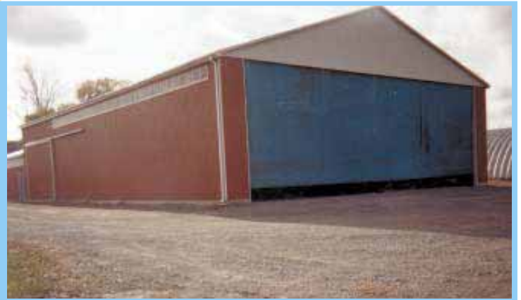
Using flexible heavy duty screening material which he got free from a paper mill, Fraser Summers built an electric roll-up door that measures 56 ft. wide by 19 ft. high.
