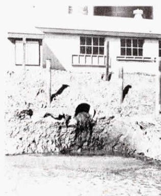
Slurry flows through 30 in. pipe from barn out of lagoon.
