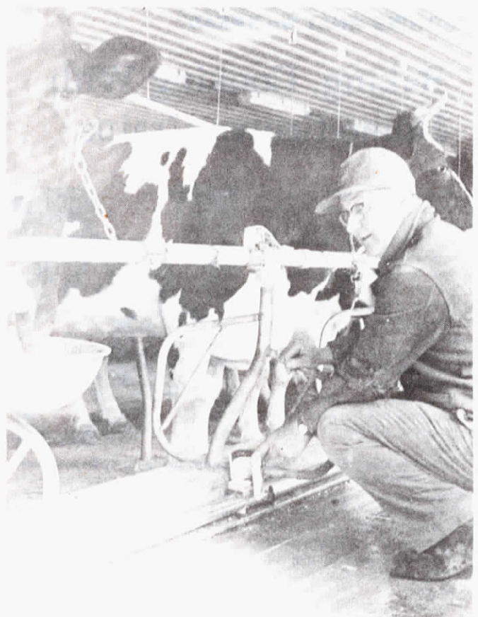
Paul Longacre lifts specially designed cover on stall cock serving his low-level milk pipeline.
