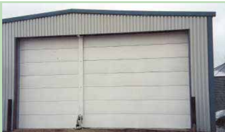
One door is 10 ft. wide and the other 16 ft. wide. Between them is a removable post that can be taken out once both doors are raised. The doors can also open independently.
