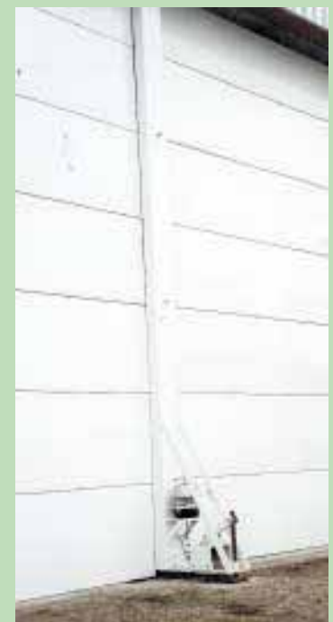
Doorpost is made from 4 by 8-in. rectangular tubing. Butuk turned the post into an air pressure tank by welding it shut.
