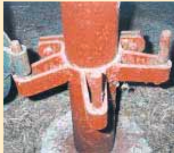
Gate hanger is designed so Kerr can lift gate off one set of hinges and replace it on one of two other sets, at a completely different angle.
