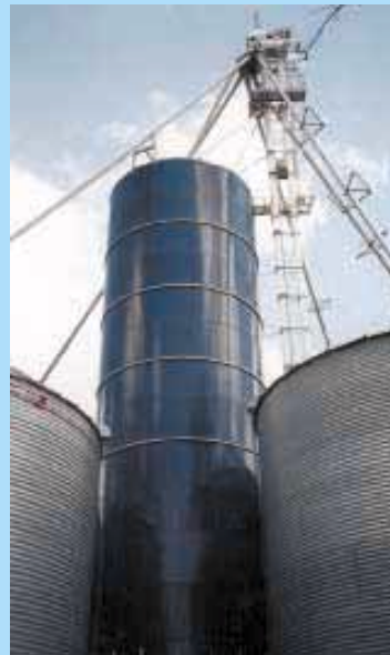
Braces run from grain leg to the top and sides of silo.
