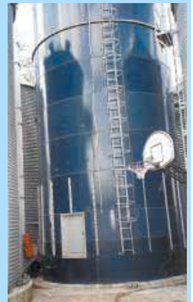
A walk-in door was installed at base of silo.
