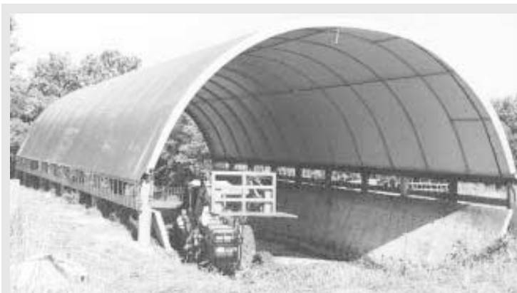
This 32-ft. wide, 96-ft. long hoop building was recently put up over a farmer's existing bunker silo.
