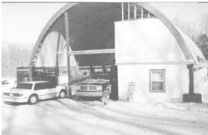
Phil Stipp, his wife and son moved into this 40 by 50-ft. Cover All building last February. They live in a 13-ft. wide area along one side of the building.
