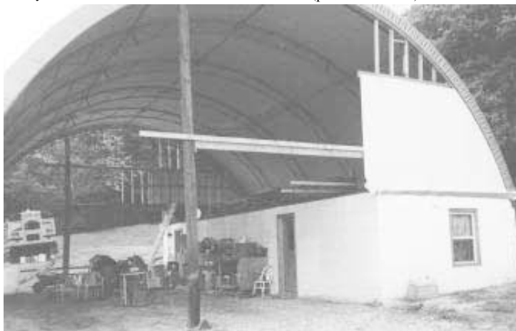
Two doors face the inside of the structure and there's a window at each end. Walls were made from 13-in. thick styrofoam blocks with hollow cores filled with concrete.
