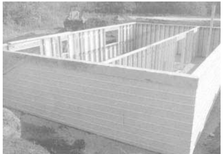
A Michigan company says it's doing a booming business in making prefabricated steel foundations like this one.
