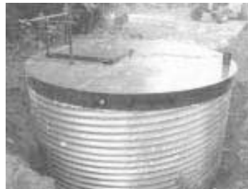
"Fraidy Hole" is an 8-ft. dia. corrugated steel pipe covered by a flat steel plate lid. It'll hold 8 people comfortably.
