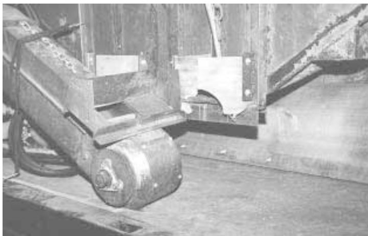
Return elevator is positioned so lower end is just below chute.
