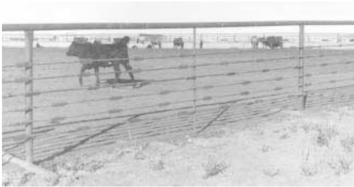
Frame of each 30 by 5-ft. panel is made from oilfield drillstem pipe while the cross-pieces are made from sucker rod.
