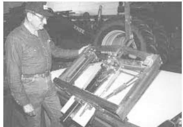
Back end of a commercial 2-in. receiver hitch bolts to center of leaf spring, cushioning the forward and backward movement of hitch.
