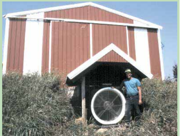
Kamps can dry up to 38 3 by 8-ft. bales at a time inside this 30 by 60-ft. building. A 38-in. dia. fan powered by a 5 hp electric motor is housed in a separate shelter alongside shed.
