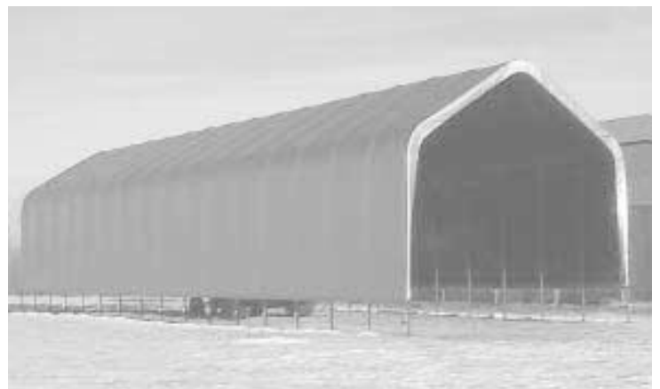
Shelter is 27 ft. wide by 96 ft. long by 25 ft. high and holds 26 typical bale wagon stacks. Roof's pitch allows snow to slide off before any accumulation can put stress on cover.
