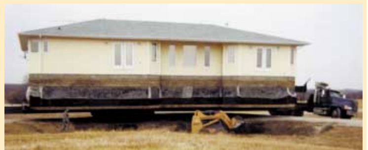
Photo shows a 42-ft. wide, 76-ft. long house with its basement on, loaded on an 80-ft. long trailer pulled by a semi tractor.
