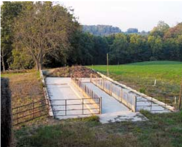
Permanent concrete feeding pads on pasture give the Sayres a place to feed big bales on a solid surface. The pads slope toward a 30 by 30-ft. manure storage pit on one end.
