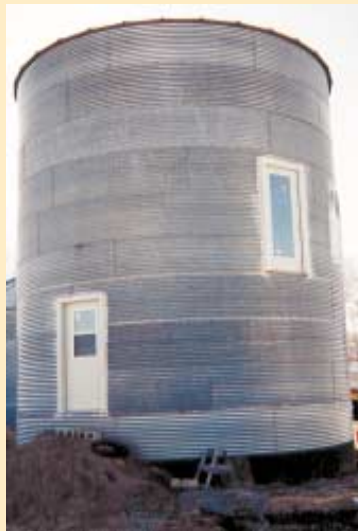
Ray Smail dismantled a pair of 24-ft. dia. grain bins and combined them into this cozy four-story home.
