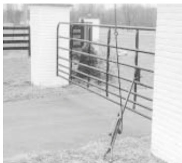
Gate from inside the fence. The toggle mechanism extends when gate is closed and folds back over itself when gate is opened. Drawing shows detail of mechanism.
