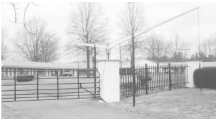
Closed gate from inside the fence. The position of the operating arms and the dangling pull chains give the gate its "grasshopper" name.
