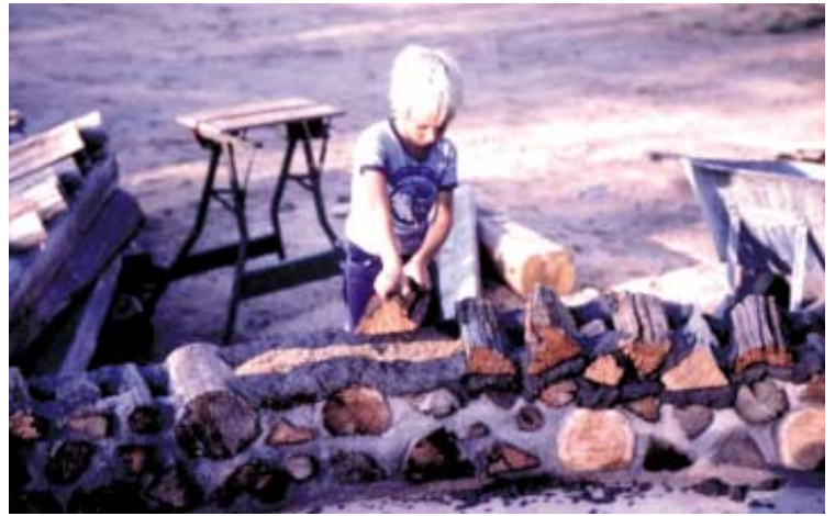
Logs of any diameter can be combined together and split wood can also be used.
