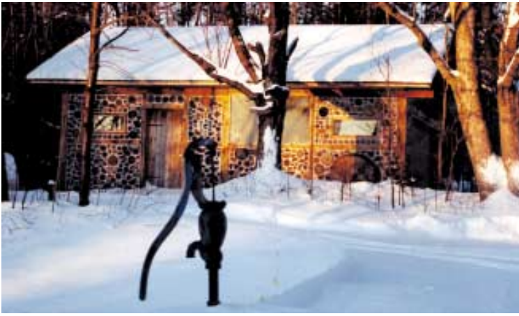
Rob and Jaki Roy built this cordwood home several years ago and now run a school teaching cordwood construction.
