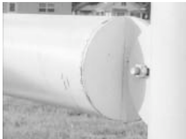
Metal tabs welded onto rails fit tabs welded onto the vertical posts. To put the fence together, you insert a bolt through a slotted hole in each tab.
