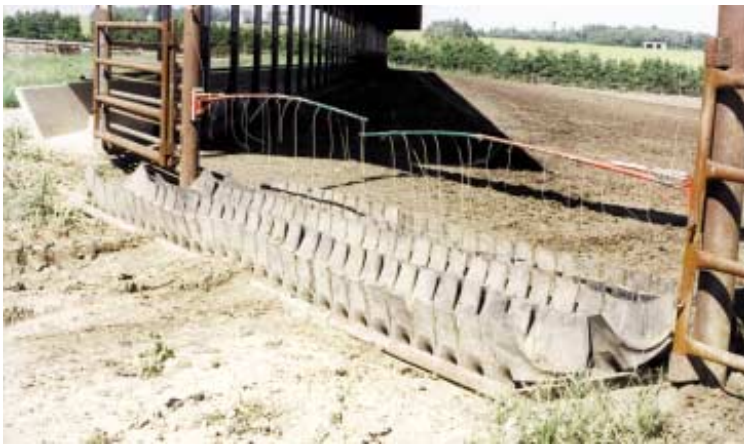
The Weitzenkamps use old tractor tires to make low-cost, drive-over cattle barriers. They're placed under drive-through electric fence gates.
