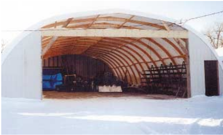
Alfred Enns came up with a process to make laminated wood "hoops" which he then covers with canvas. He says wood is cheaper than steel.
