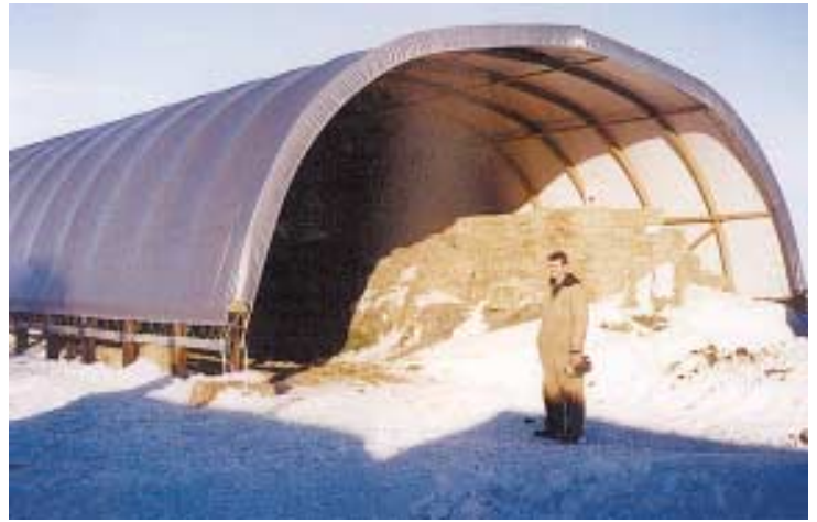
Beams are 8 in. deep so building can be easily insulated. Wood frame makes it easier to replace the canvas cover with wood or metal siding at a later time.
