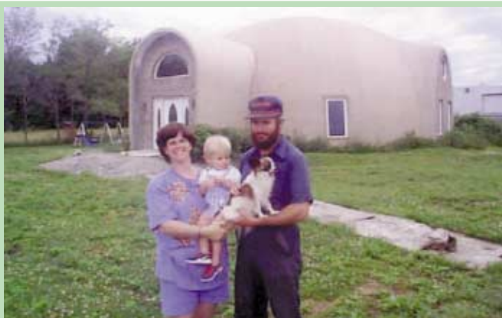
Cindy and Lee Quaintance have built one of the only monolithic dome homes in the country. It's 53 ft. in dia. and 24 ft. at the peak, making it "look sort of like an igloo."
