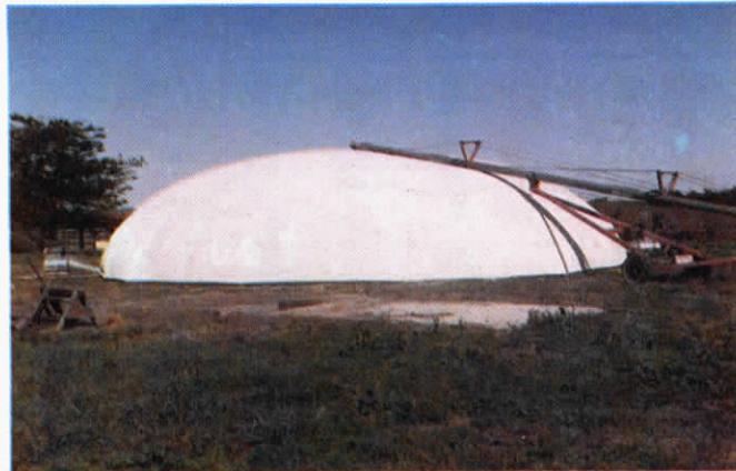
“Air Bubble” bin holds 6,000 bu. It's inflated by a blower system that also serves as a grain aerator.
