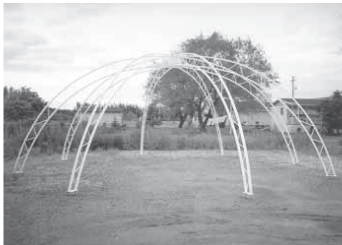
Photo shows first prototype of Silver Stream's new "hooped dome" building.
