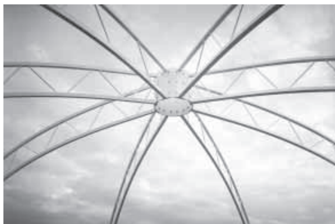
Steel trusses meet at a central hub. Buildings are available in diameters ranging from 30 to 50 ft.
