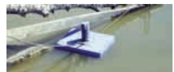
Pump is tied to a stake to keep it in place.
