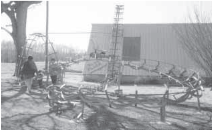
John Ivers built this roller coaster in his back yard. It measures 180 ft. long, 20 ft. high, and goes up and over the barn behind his home.
