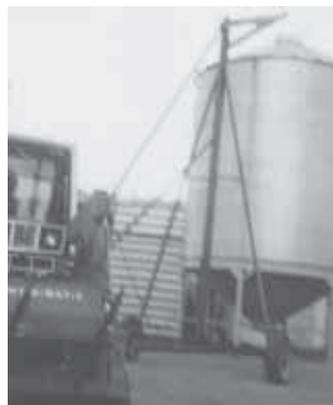
Husak also built a hydraulic-operated, two-wheeled bin crane.
