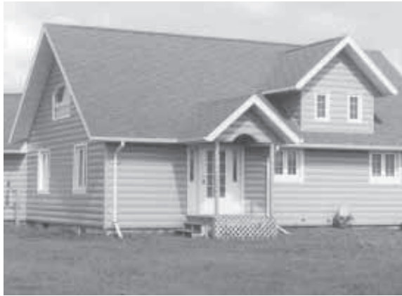
Steel siding is formed in the shape of a log or half log. It's available in 15 different colors.
