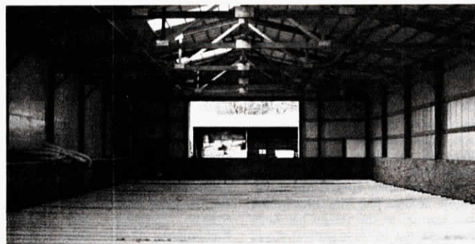
Air is distributed by perforated 4 in. dia. plastic drain tile spaced 6 in. apart under grain.
