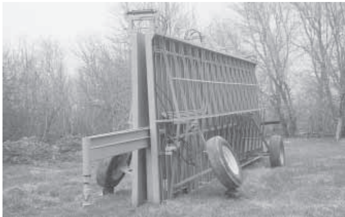
Portable "form" creates a 10-in. thick free-standing wall.
