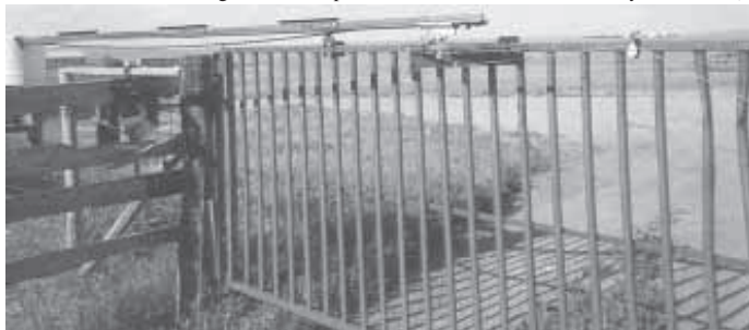
Pivoting bracket mounts on top rail of gate. Garage door opener "carriage" attaches to bracket.
