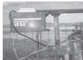
Egli mounts the motor and track on a post 2 ft. from fence and 2 ft. behind the post holding gate.
