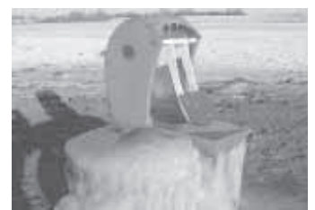
Geothermal heat, in combination with an insulation sleeve, prevents freezing.
