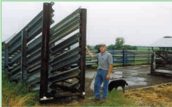
Farley Cole used highway guard rail to build a loading chute and a corral that measures 30 ft. wide by 60 ft. long.
