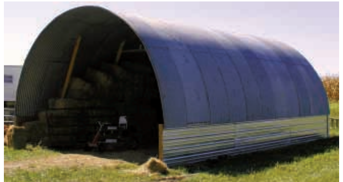
Brent Brueland took down a 5,000-bu. grain bin piece by piece and converted it into this 20 by 30-ft. hoop building. It mounts on two 3-ft. tall "knee walls".
