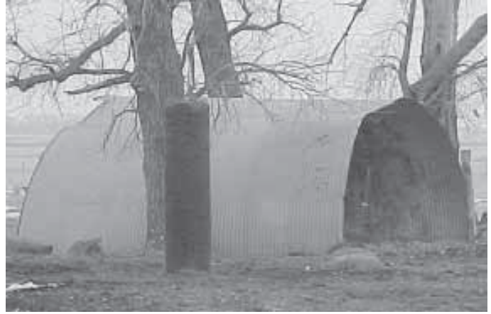
Braton cut a couple of empty grain bins in half to make two quonset-like sheds that are open at both ends.
