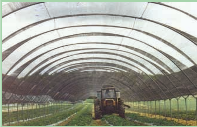
Haygrove tunnels have metal frames covered by plastic that can be rolled up on the sides. Units come in widths from 18 to 27 ft. and can be built to any length.
