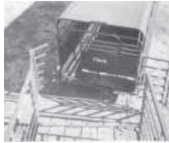
Livestock chute is fitted with a bi-fold gate on either side. Each gate is built in two sections. Hinges at top and bottom allow gates to be folded completely to either side.
