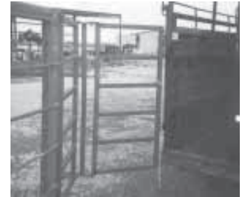
Livestock chute is fitted with a bi-fold gate on either side. Each gate is built in two sections. Hinges at top and bottom allow gates to be folded completely to either side.
