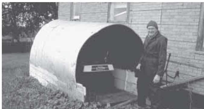
Ray Obrecht positioned two hog feeders end-to-end to make this low-cost shed.
