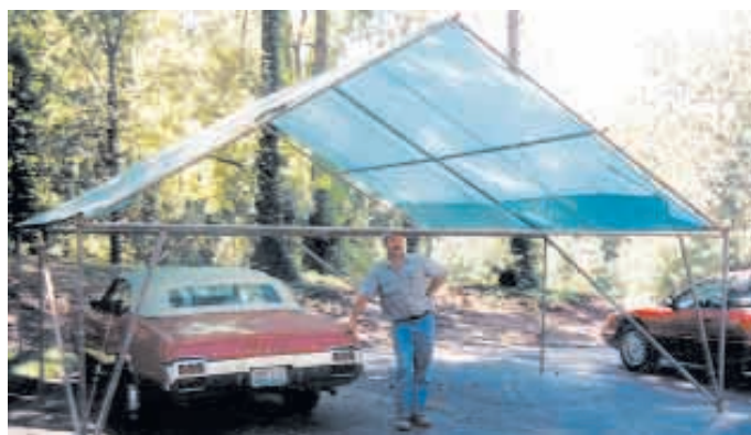
Car shelter is made out of gas pipe covered with a plastic tarp.
