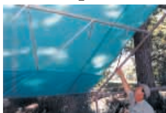
Elastic straps run from mid-mounted pipes on each side to ends of tarp, which folds under edges of roof.
