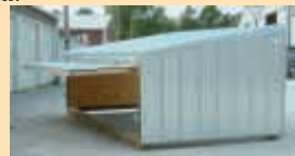
Hog pasture shed has galvanized metal sides with an open front and no floor. Back side is hinged at top and can be opened for ventilation.
