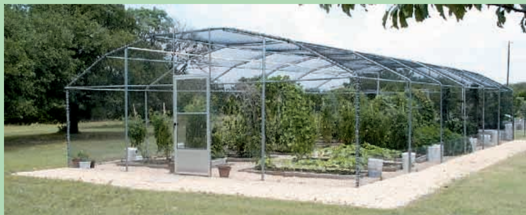
To make this gardenhouse, Janet Willie simply covered a greenhouse frame with bird netting and added doors.
