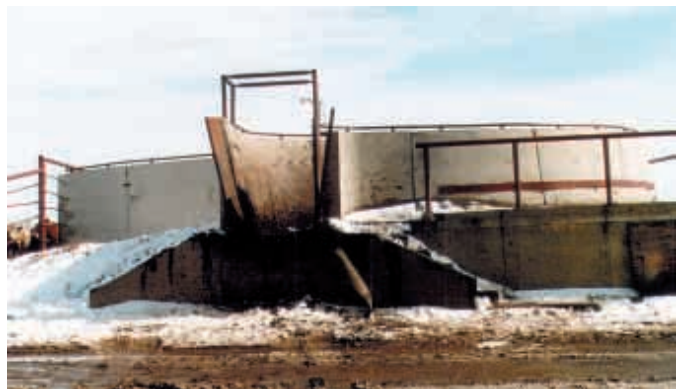
Walls on concrete tub are about 5 1/2 ft. tall and limit the view of animals inside. A steel rail along top is safety precaution, giving workers something to grab onto.
