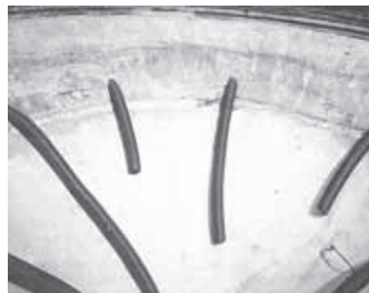
Above photo shows aeration tubes that extend down into cone. Elevator leg next to bin, right, carries grain to dryer.
