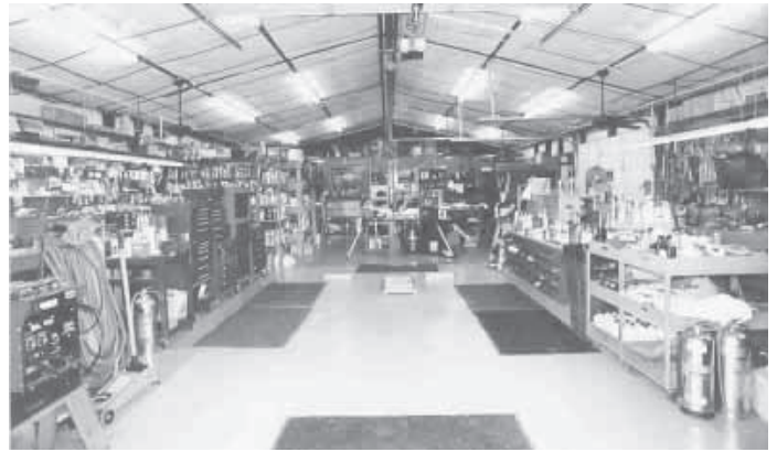
To create the "guest house" living quarters, Yager put up a wall 12 ft. from one end of building and across the full 30-ft. width of it.
