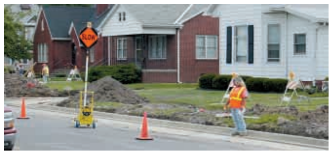
Riding on wheels, flagger consists of an upright sign that says "stop" on one side and "slow" on the other, with a flashing light above. A hand-held controller connects to flagger by an electric cord.
