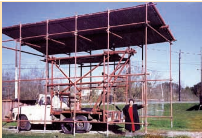
You can use all kinds of steel pipe to put up building frames with new clamps designed by Mills Tourtellotte, Rosenberg, Texas.
