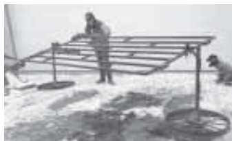
Stand is used to rotate gate like a paddle wheel, which eliminates the need to do any lifting.
