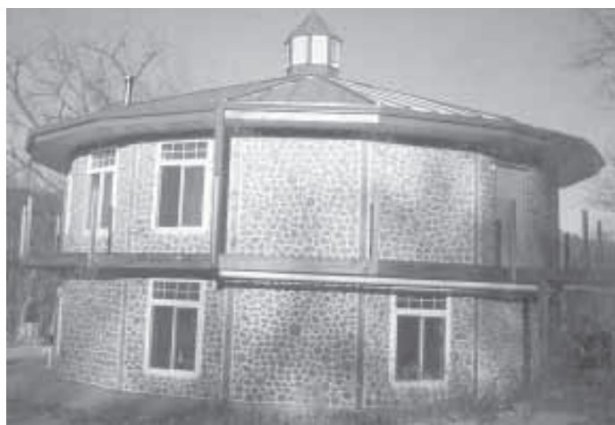
More than 6,300 8-in. lengths of cordwood form the walls of the post and beam-framed house built by Alan Stankevitz near La Crescent, Minn. The cordwood is set in mortar that has newspapers mixed into it.
