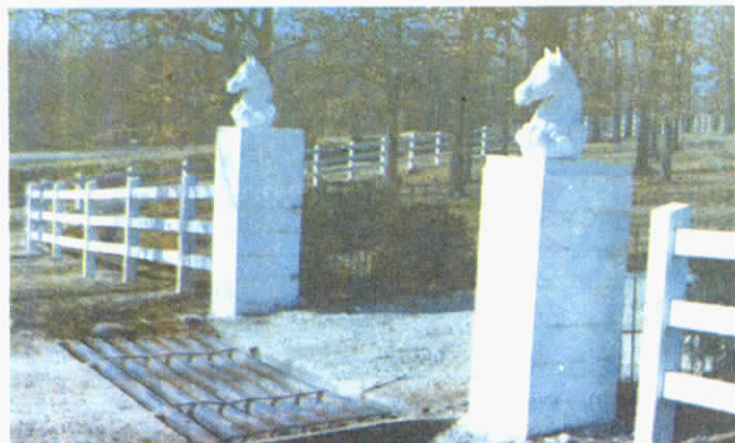
The special concrete can be colored as it's mixed, or painted after fence is up.
