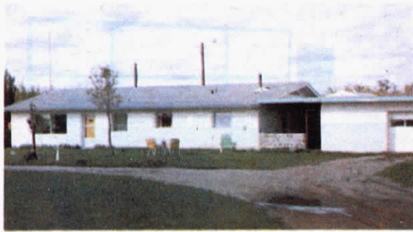
Stucco, both inside and out, covers rammed earth walls of the Larson home.
