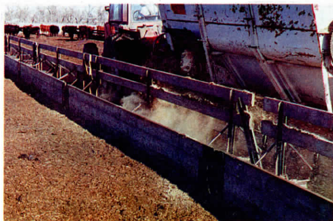
Feeders have wood planks held in place by channel iron and internal cross braces.
